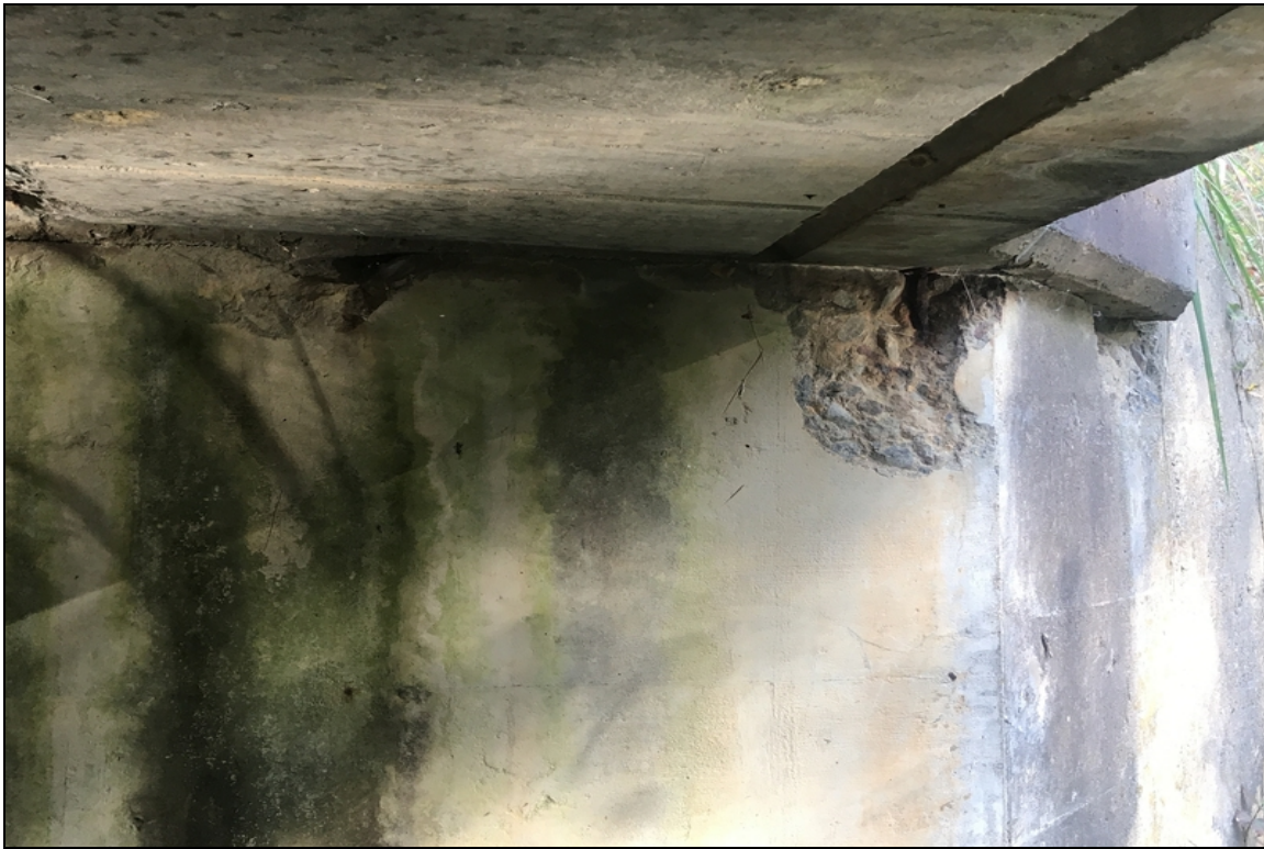
Bent 2 abutment has spall with exposed rebar.
