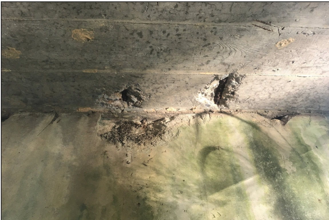
Soffit has spalls with exposed rebar near bent 2.
